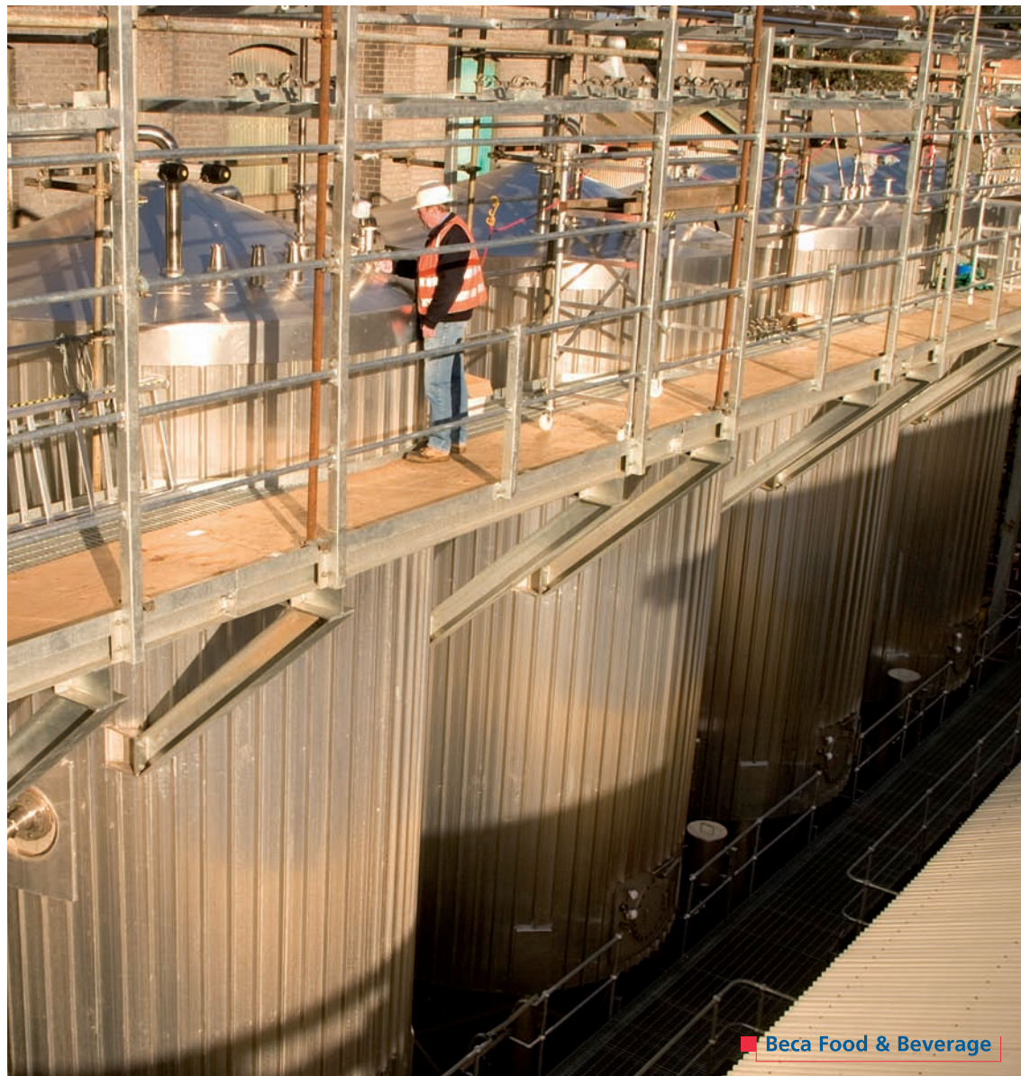
Key refinery upgrade for Sugar Australia (see story on back cover)
