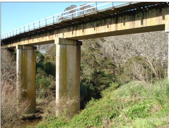
Photo 3 – Typical KRN concrete bridge
