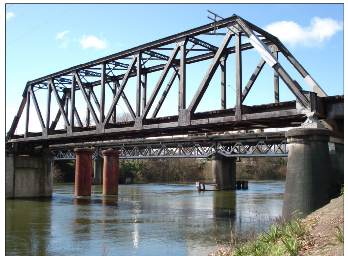
Photo 1 – Typical KRN steel truss bridge
