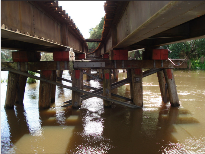
Photo 2 – Typical KRN steel bridge with timber piers
