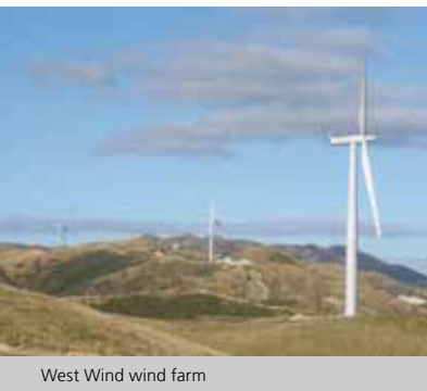
West Wind wind farm
