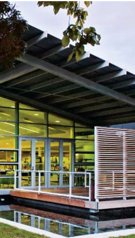
South Christchurch Library & Community Centre // Christchurch
