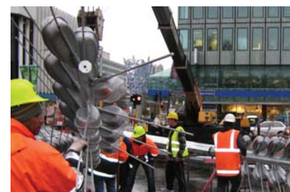
Erecting Flour Power, Regan Gentry Photo: Fletcher Construction
